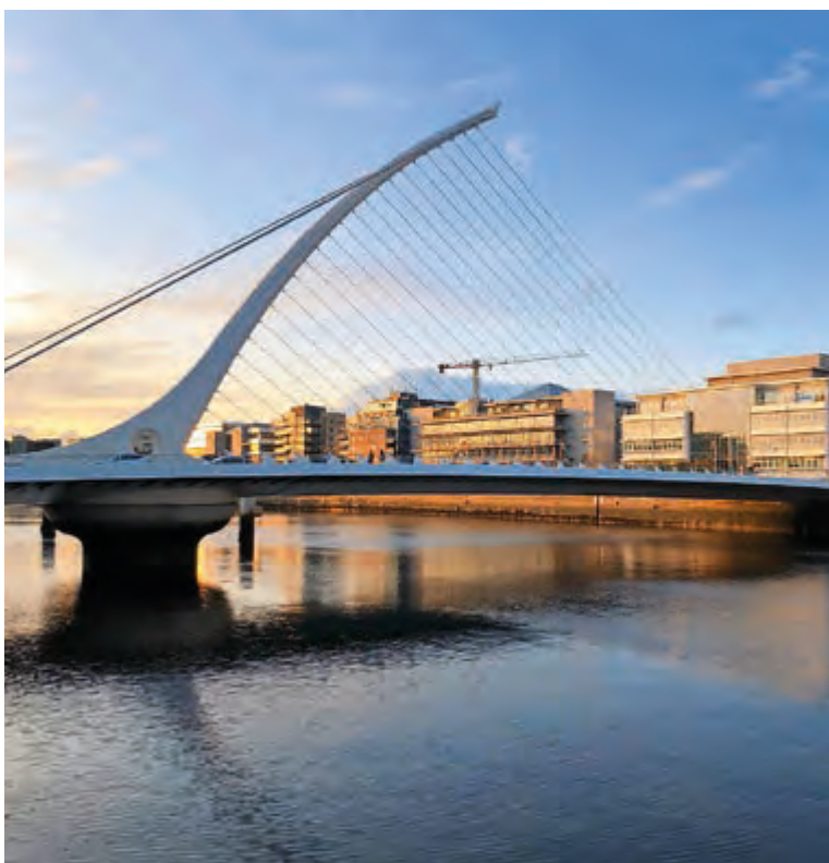
Die Samuel Beckett Bridge in Dublin.
