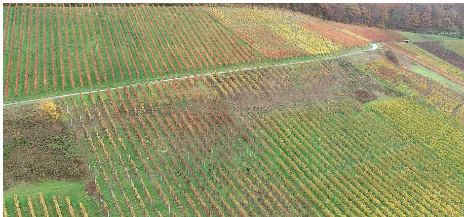
Fig. 2: Visible break-off edge (Drone image by Heilbronn Surveying office)
