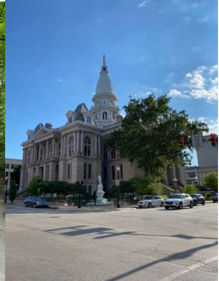
Court House in Downtown Lafayette
