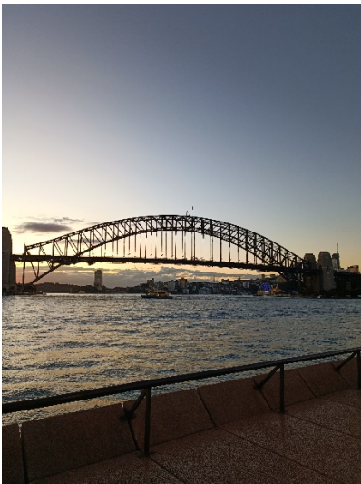
Sydney Harbour Bridge
