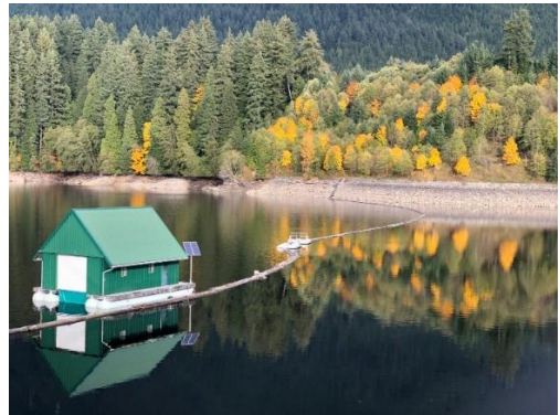
Cleveland Dam, North Vancouver
