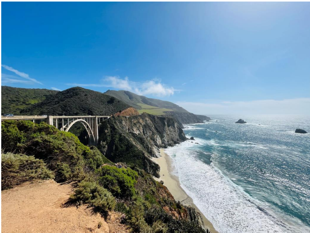
Abbildung 3: Bixby Creek Bridge am Highway 1
