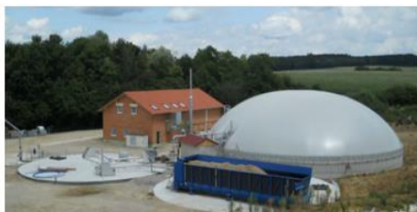
Bio gas systems
