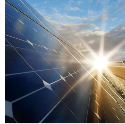
Solar Technology and Electrical Power Systems
